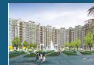
Harmony @ Jaipur-ajmer expressway, Jaipur
